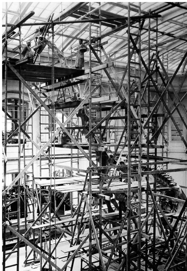
**FIGURE 18.2.** The mount of *Brachiosaurus brancai* shortly before completion in late 1938. The ribs had not yet been mounted at the time the picture was taken. Note the extensive wooden scaffolding and the still-uncolored plaster models of the presacral vertebrae.
